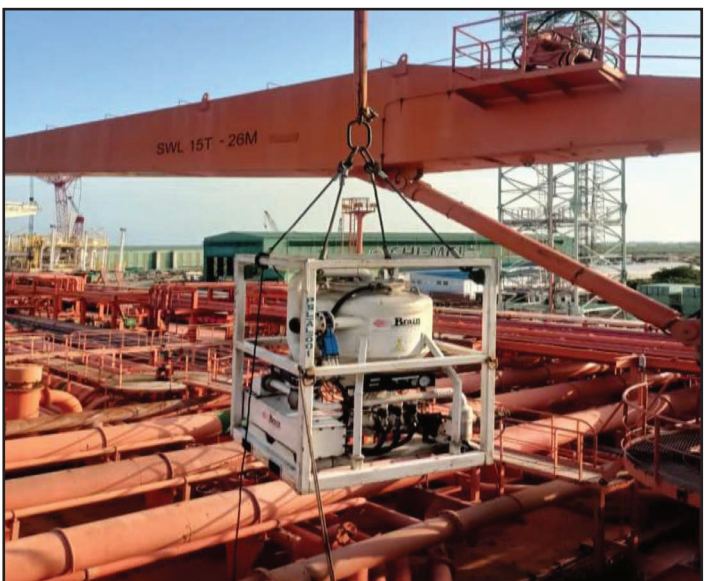
Air Loader Pump Being Set onto FPSO
