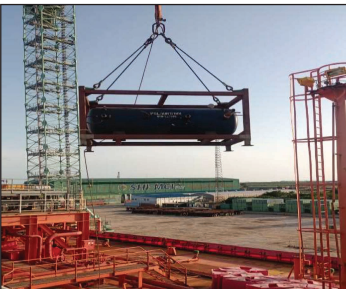
Air Tank Being Hoisted onto FPSO
