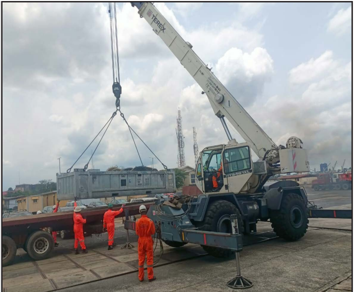
SWDA Hose Basket Hoisted onto FPSO
