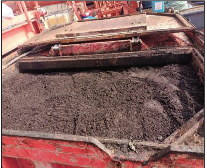
Solid Sludge Removed & Stored in On-Site Waste Skips on FPSO
